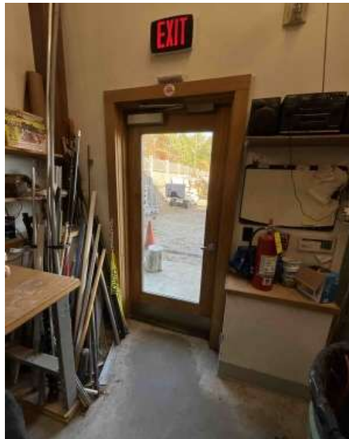
Garage exterior exit door
