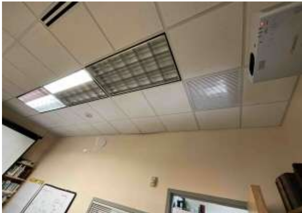
Conference Room ceiling
