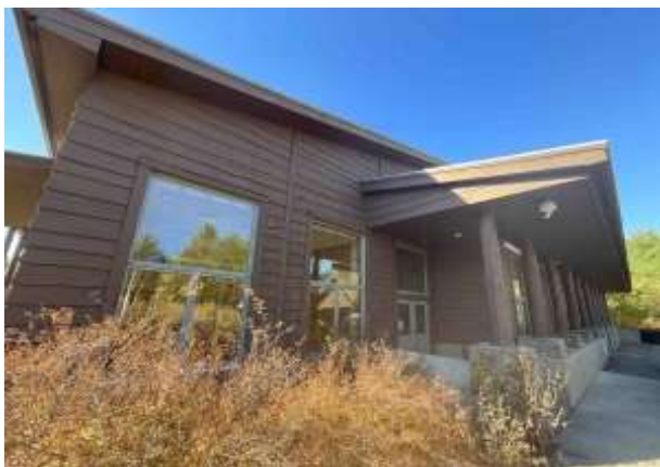
Conference/Admin entrance of Museum Building
