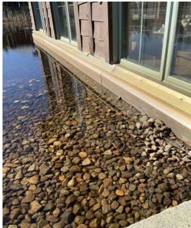
Figure 8 Pond Liner at Building Foundation
