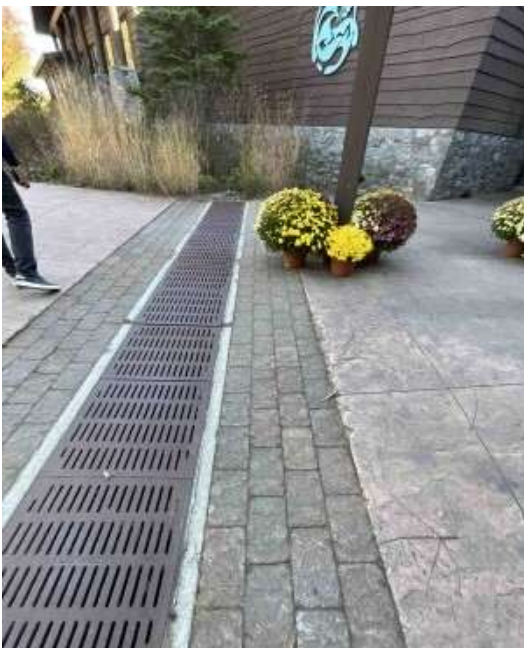
Figure 1 Stormwater drainage near building front entrance
