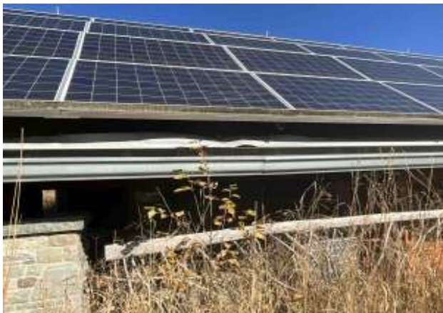
Roof flashing at solar panel locations
