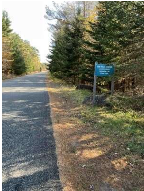
Figure 3 Entry signage, good condition, vegetative management recommended
