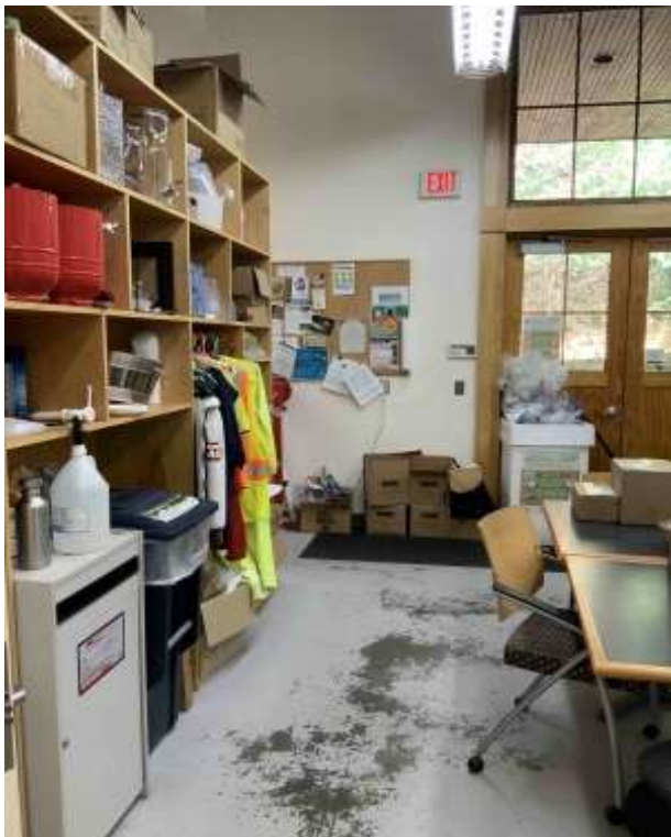
Examples of concrete floor requiring refinishing or repair
